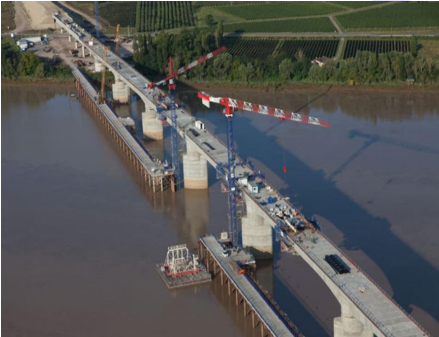
Photograph of a new bridge under construction near Bordeaux Credit: 20minutes.fr
