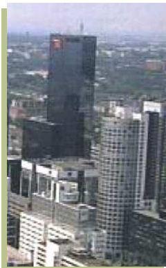
R'DAM NN 35 FLOORS 150 m Concrete
